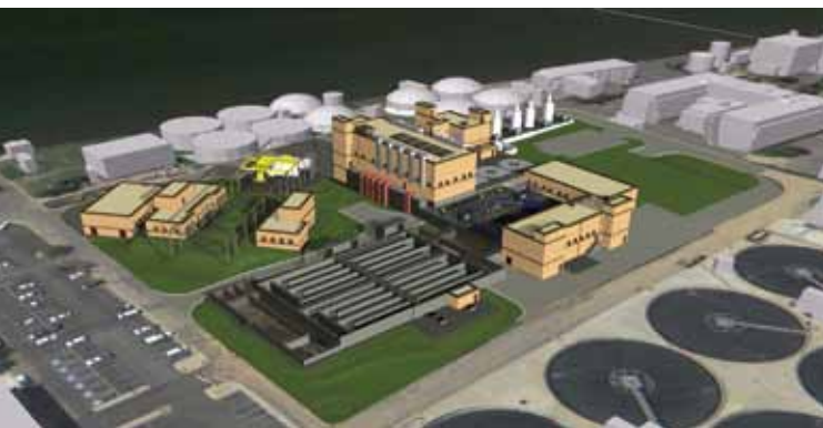
Combined sewage will be captured, stored and conveyed for treatment at the Blue Plains Advanced Wastewater Treatment Plant.
