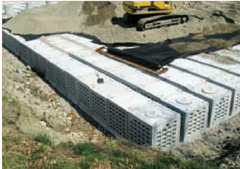
Underground storage options include “box of rocks,” rectangular tanks and chambers; and stone with embedded chambers.
